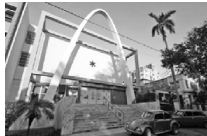
Havana's renovated Patronato Synagogue and JCC houses a library, social hall, classroom, youth center, computer room, and the community pharmacy.
